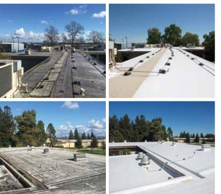
Roofs restored with AlphaGuard<sup>™</sup> BIO reflect the sun for lower energy use.
